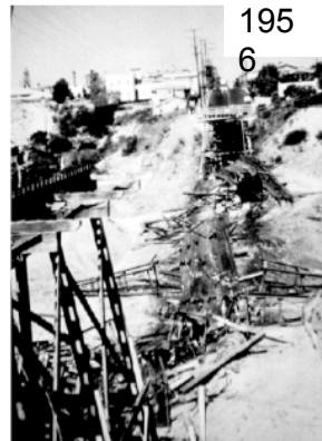
The 1956 demolition of the original trolley bridge.
