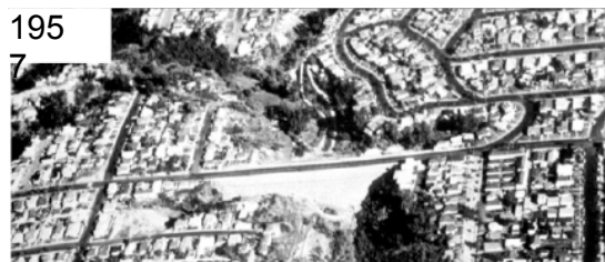
Aerial view of the 30th St. replacement landfill bridge at Switzer Canyon.
