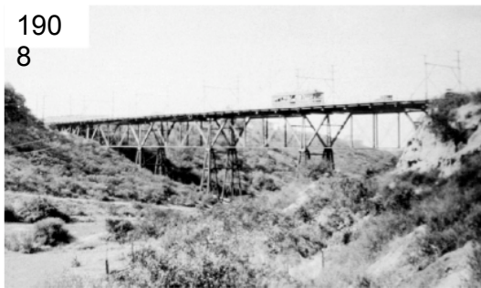
Canyon view of the original steel and wood 30th Street trolley bridge.
